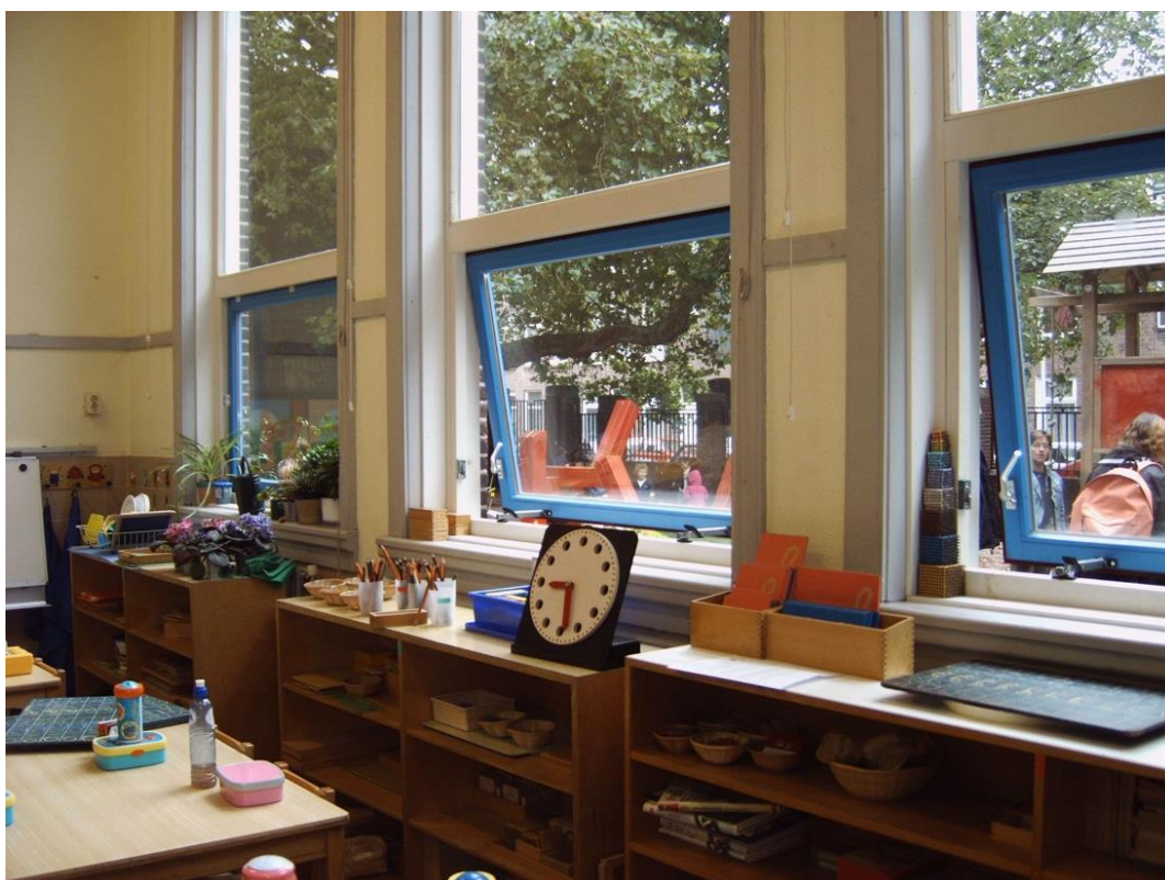
Figure 18. Open windows as much as possible during school hours and ensure airing during breaks.
